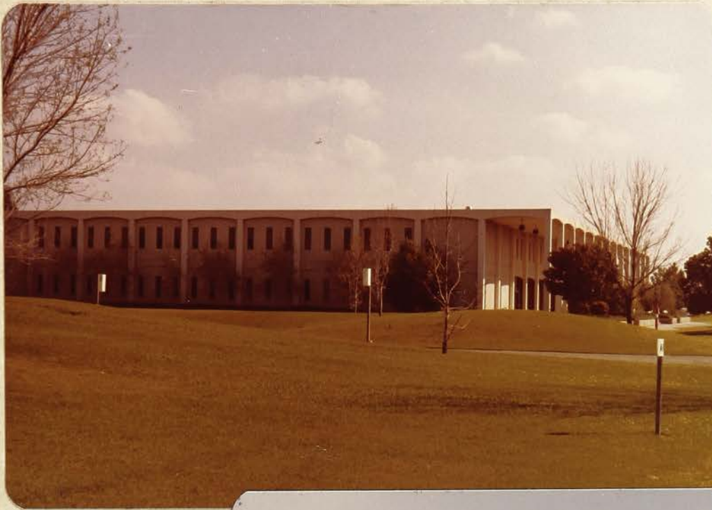
This is the Joyal Administration Building. It is located on Maple Avenue
