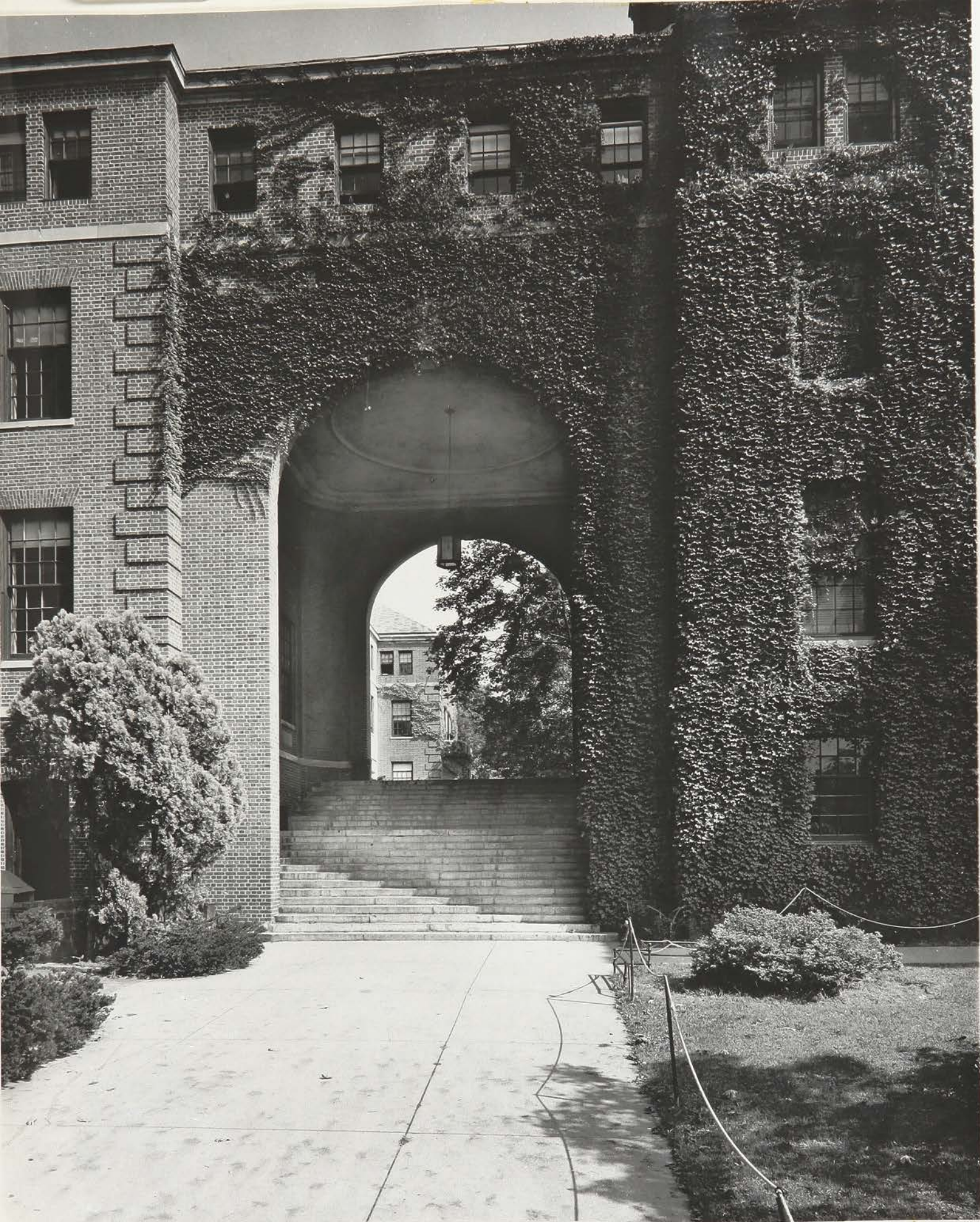
West Archway of Quadrangle De La Salle Hall on Left
